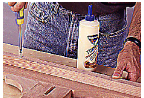
6--When leg/bracket assemblies are finished, join them to the rails. Apply glue to plate and mortise-and-tenon joints, then clamp.
